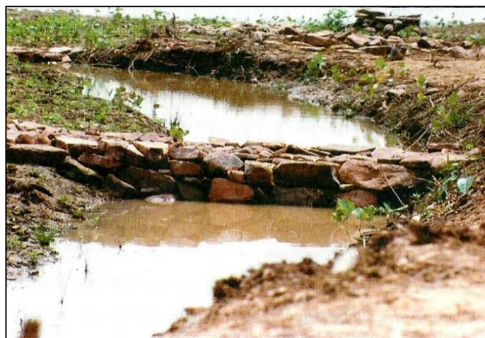
loose boulder check dam at Chitauriha
