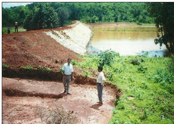
A side spillway at zero level, trenches at Khodari village.
